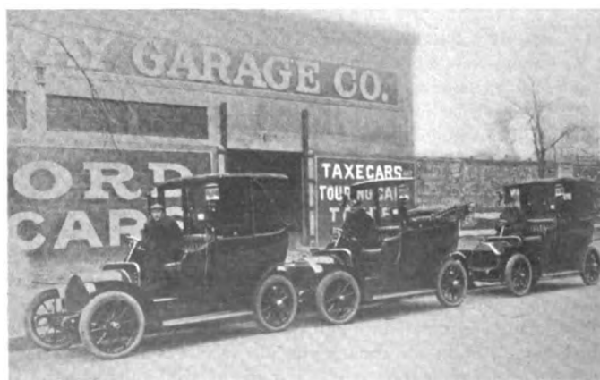
Parkway Garage, at 110th Street, New York City.
